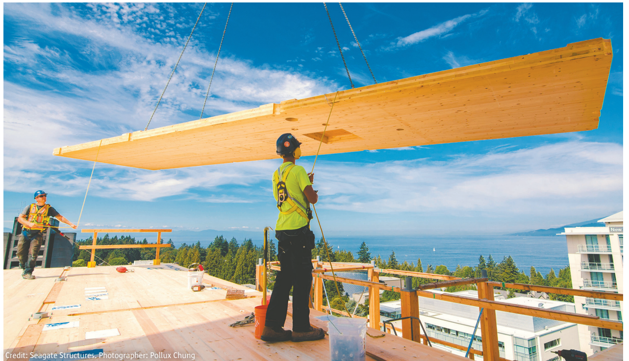
Credit: Seagate Structures. Photographer: Pollux Chung Balanced CLT panel lift
