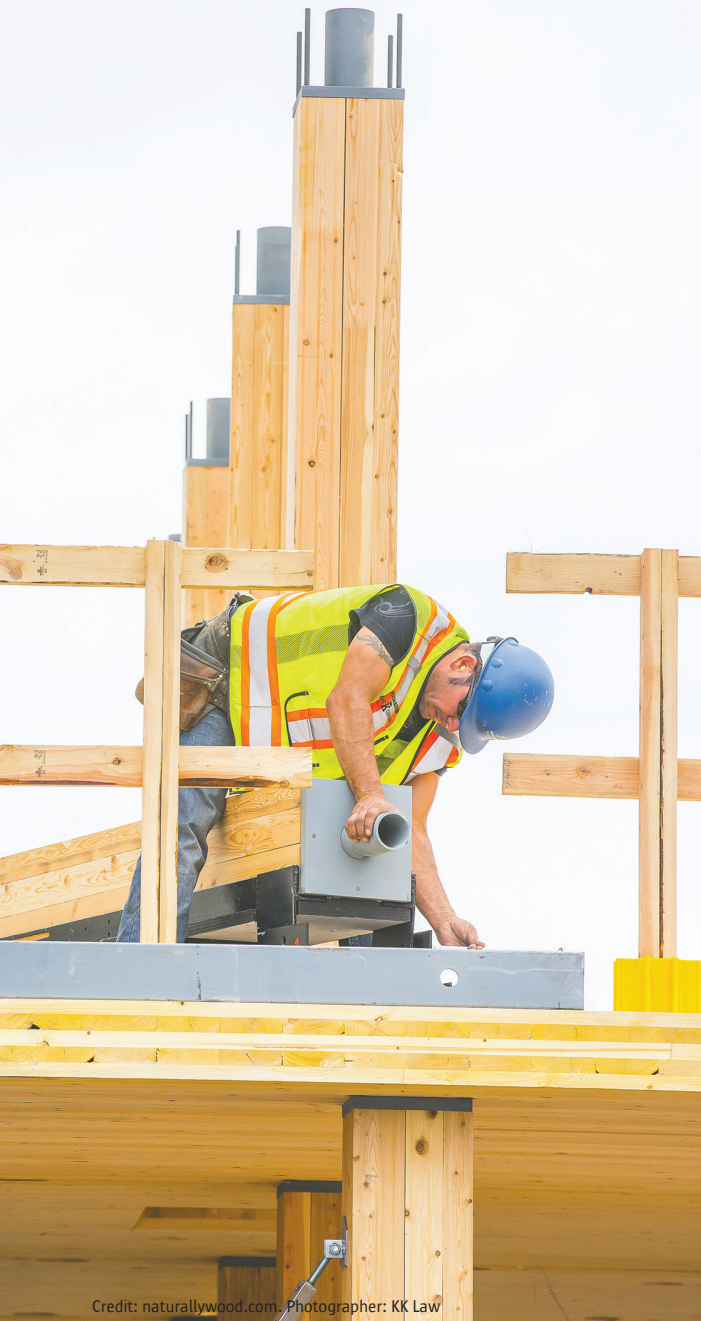
Glulam column installation
