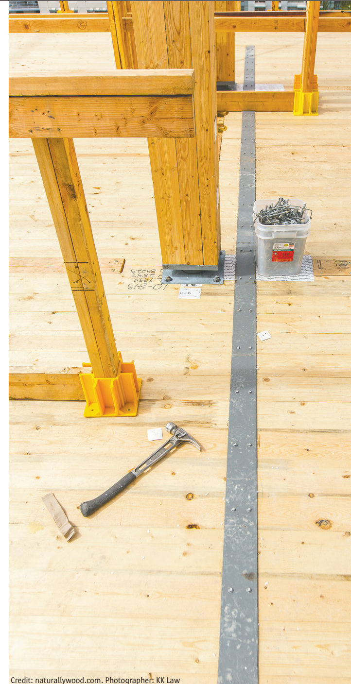
Credit: naturallywood.com. Photographer: KK Law Drag staple connecting CLT floor panels and reinforced concrete core
