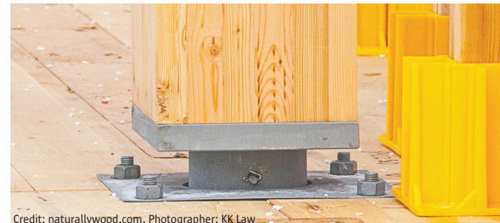
Credit: naturallywood.com. Photographer: KK Law Column-to-CLT slab detail before concrete topping
