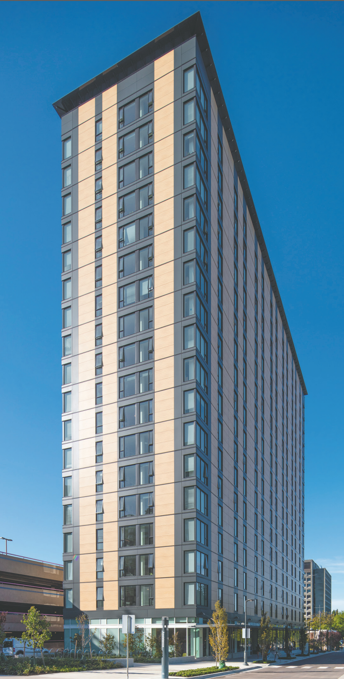
Credit: Acton Ostry Architects & University of British Columbia. Photographer: Michael Elkan Brock Commons Tallwood House
