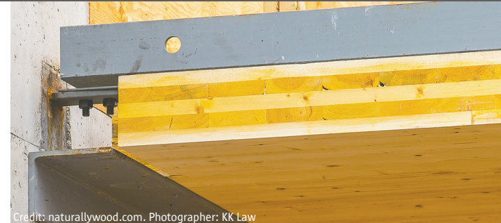
Credit: naturallywood.com. Photographer: KK Law Drag strap and angle iron connection to the reinforced concrete core
