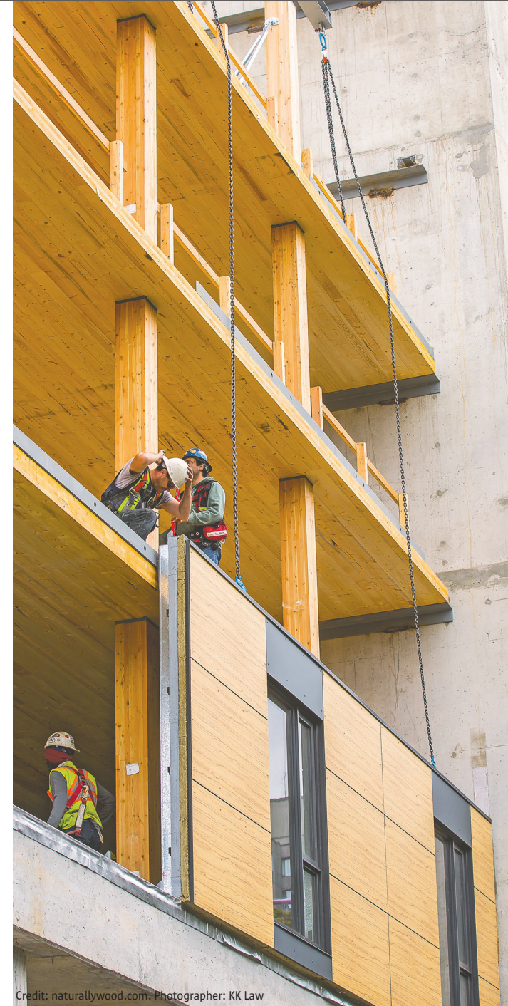
Building envelope panel installation
