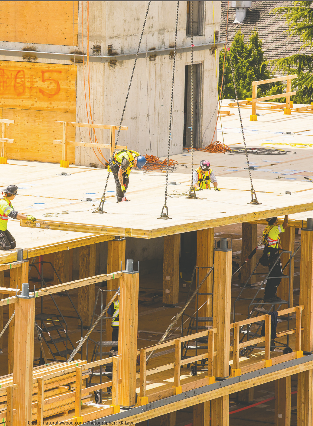
CLT panel installation
