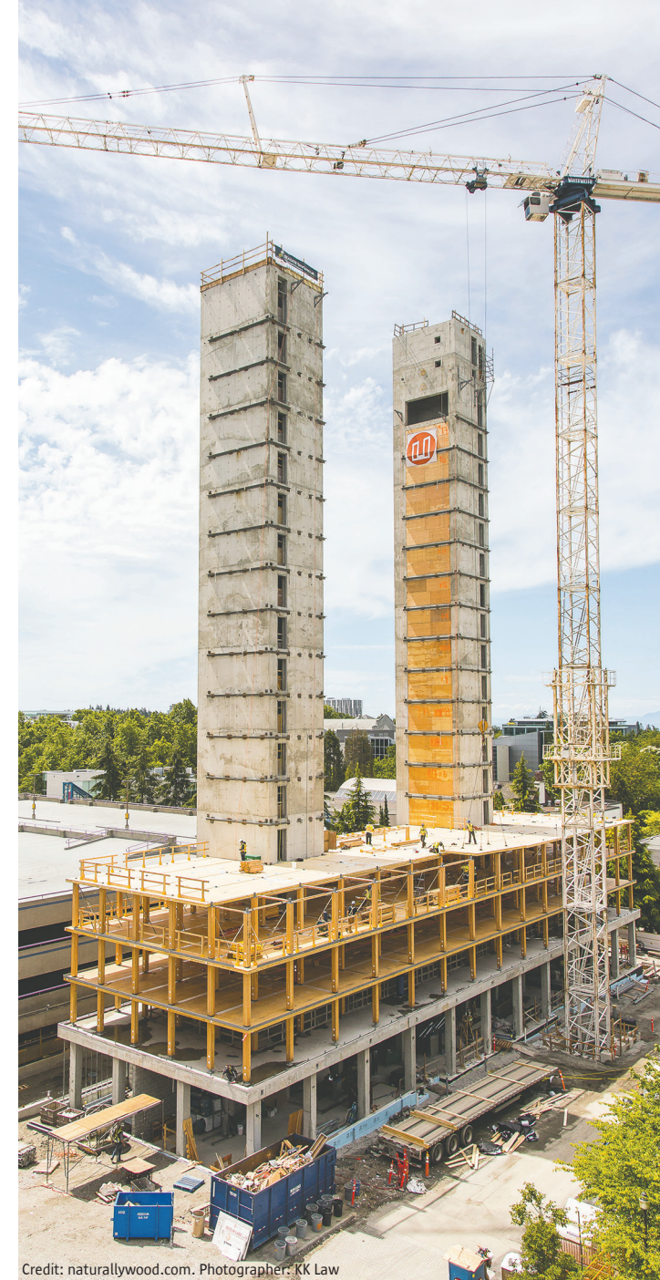
Credit: naturallywood.com. Photographer: KK Law Under construction – Late June 2016
