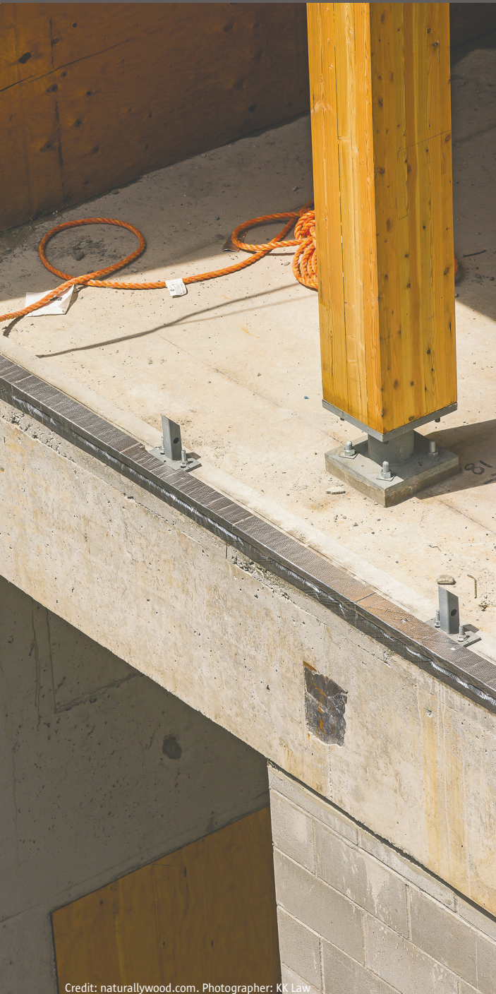
Credit: naturallywood.com. Photographer: KK Law Column and building envelope connection detail at transfer slab
