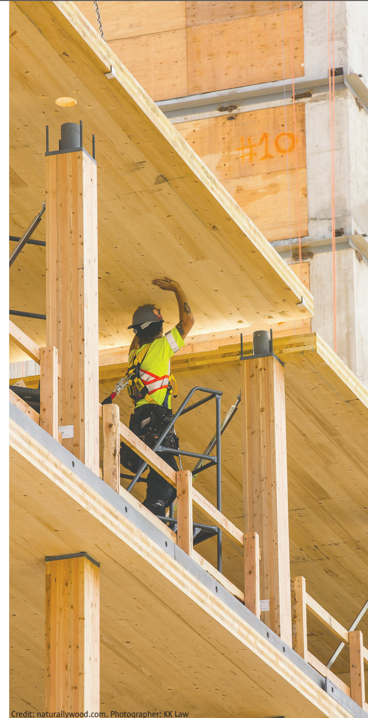
Credit: naturallywood.com. Photographer: KK Law CLT panel installation
