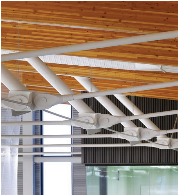
Arena truss connections
