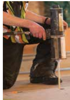
Epoxy injection for securing the HSK plate
