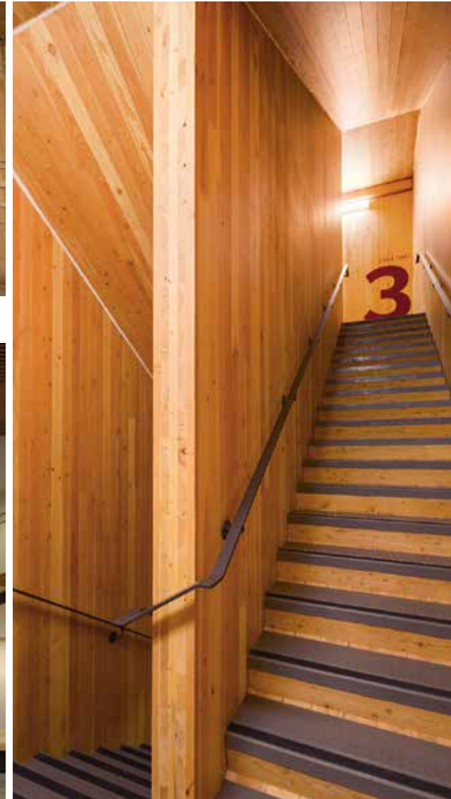
Stairwell with CLT walls, ceiling and floor
