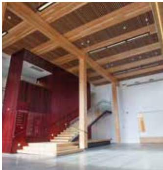
Ceiling cavities in the Level 1 demonstration area contain lighting and fire suppression systems concealed by a removable wood-slat finish
