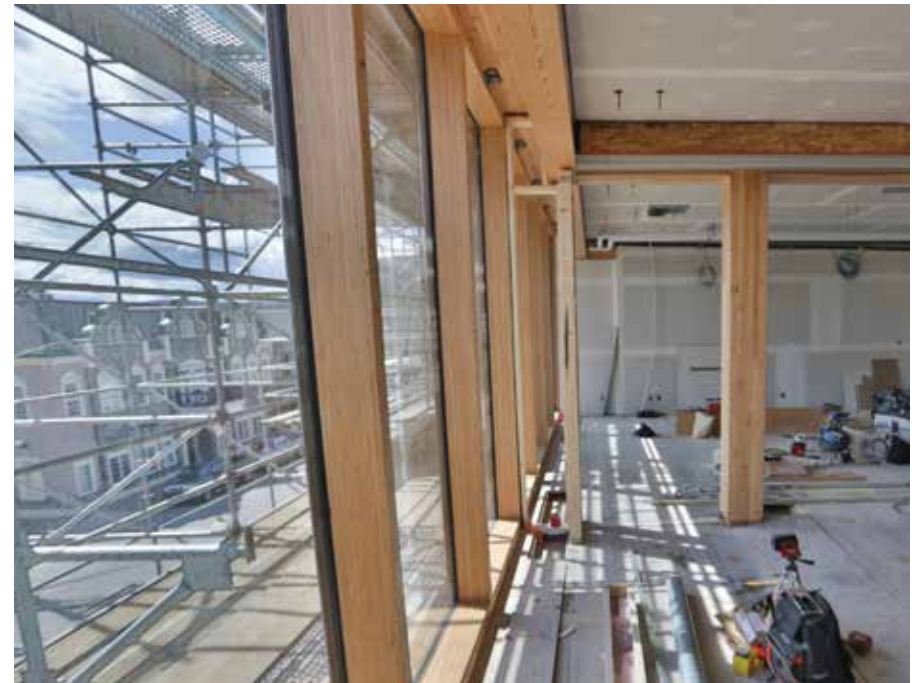
Window mullions after glazing installation
