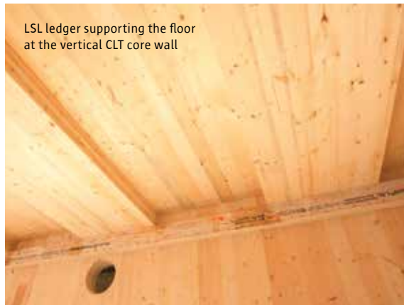
Self-tapping screws readied for attaching a ledger to the CLT core
