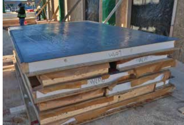
SIP panels with air barrier membrane on the exterior face
