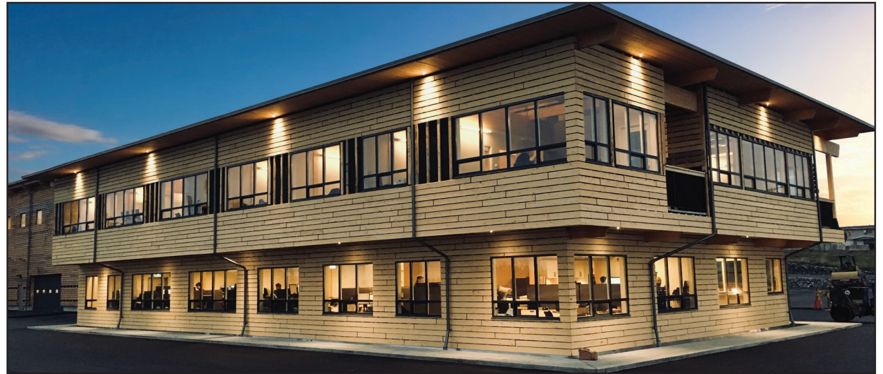
Fig. 4.13: Exterior of office building
