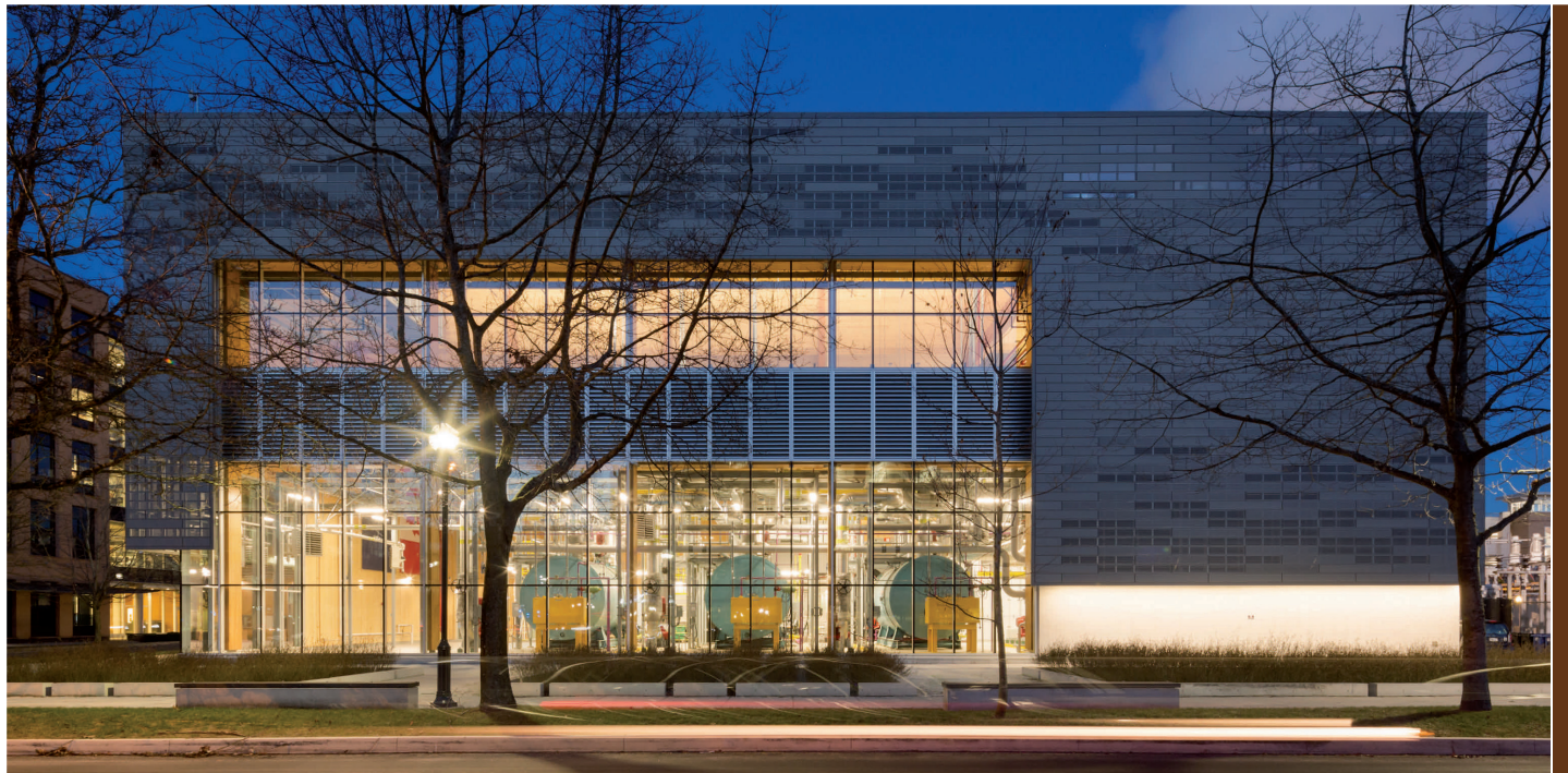
Fig.3.1: UBC Campus Energy Centre
