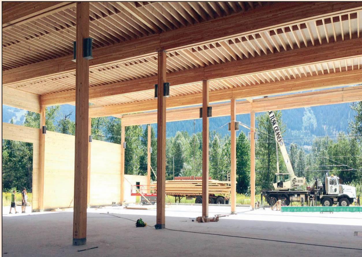
Fig. 2.9: The central line of columns reduces the depth and cost of the roof structure
