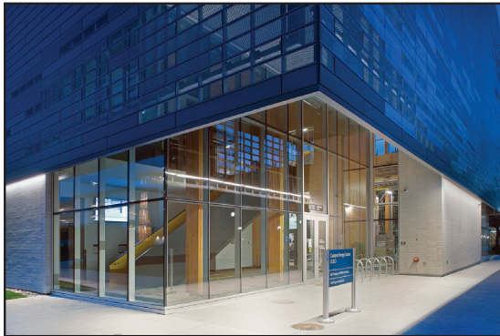
Fig. 3.7: The exterior zinc screen rises at the corner to reveal the main entrance
