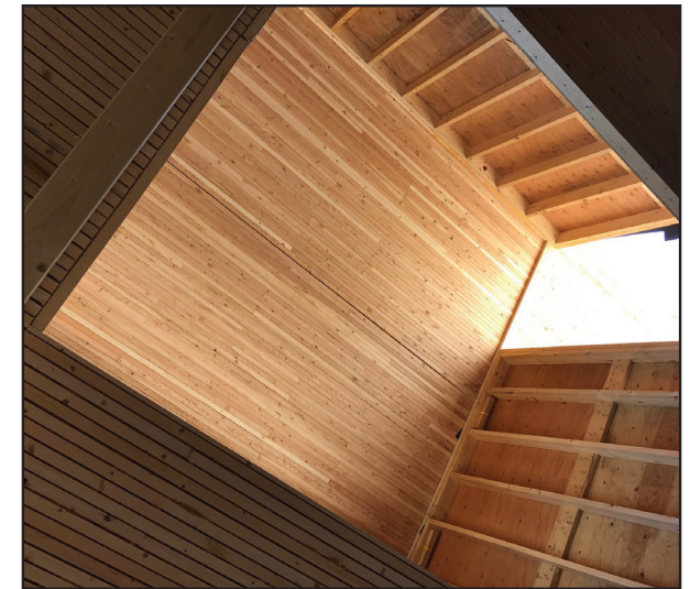
Fig. 4.15: Feature wood stair in the office area
