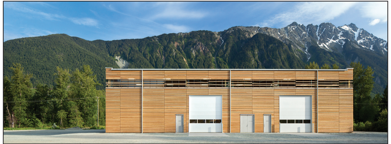
Fig. 2.6: BCPH sets a new standard for the design of industrial buildings
