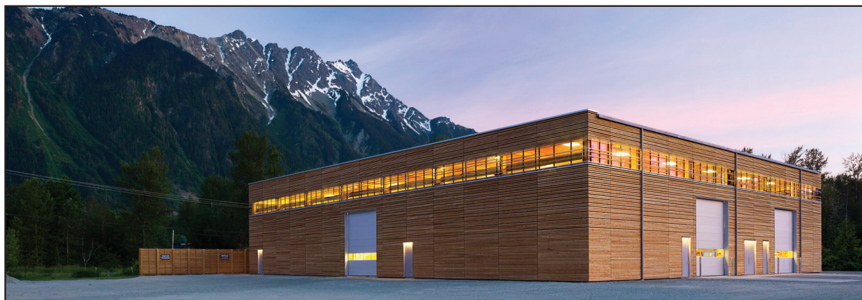
Fig. 2.15: The building itself is an advertisement for the advanced wood components made within
