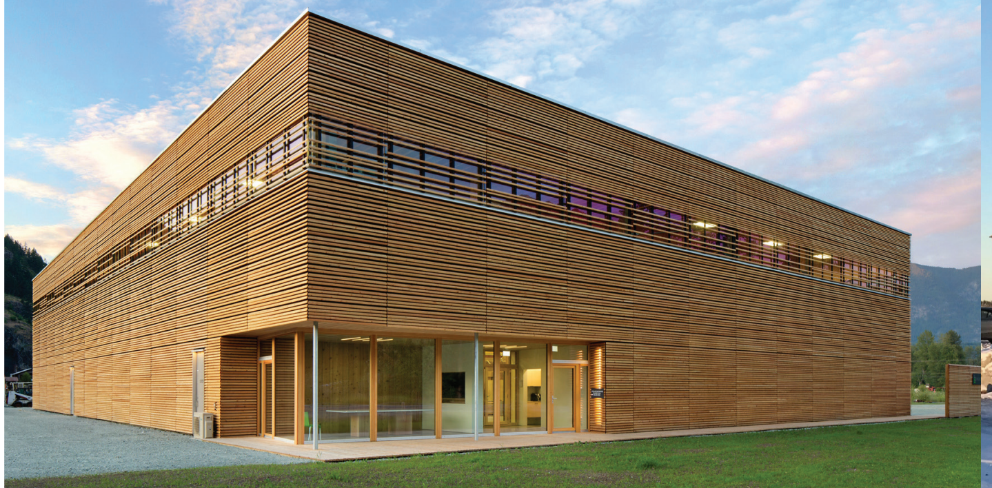
Fig. 2.1: BC Passive House Factory
