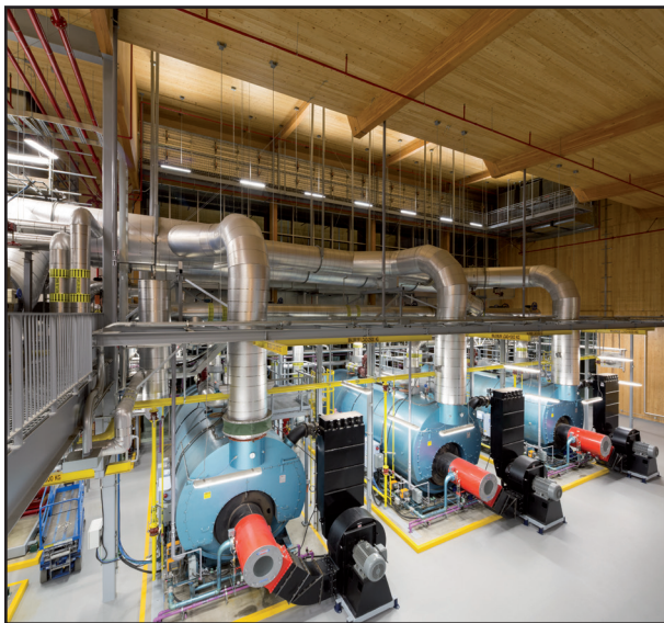
Fig. 3.4: View of boiler bay from mezzanine
