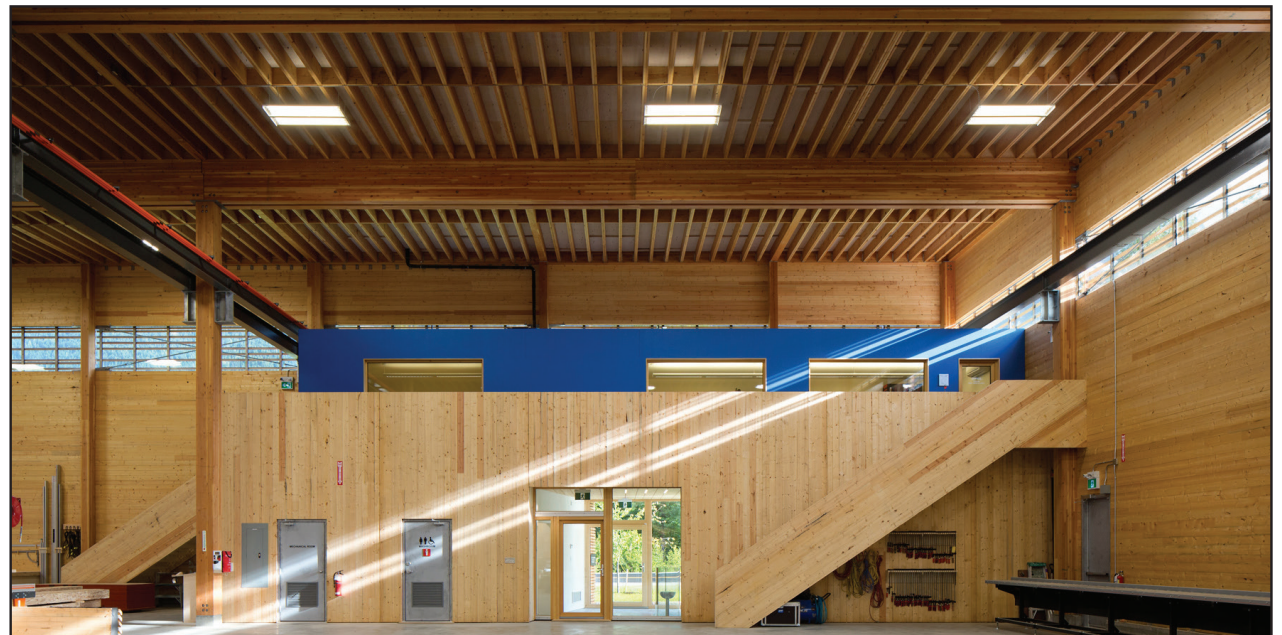
Fig. 2.7: Abundant daylight and exposed wood finishes give the interior a warm and inviting quality
