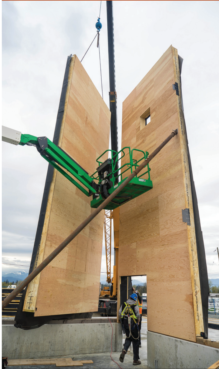
Fig. 4.5: Wall panel being placed
