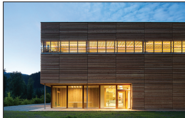
Fig. 2.3: The showroom and office areas are constructed to the Passive House Standard
