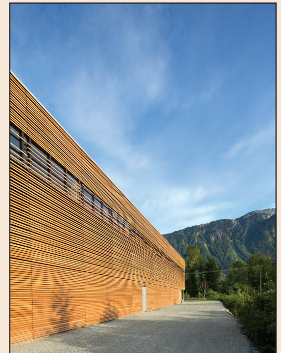
Fig. 2.14: The wood cladding is left unfinished, and will weather to a grey colour over time
