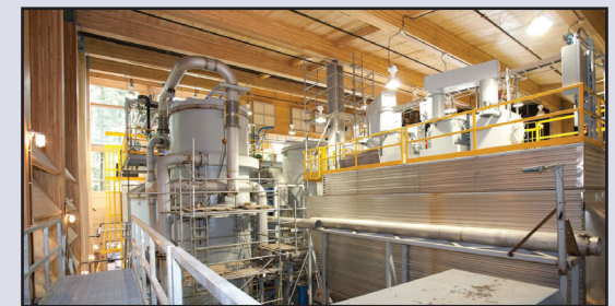
Fig. 3.3: The UBC Bioenergy Research and Demonstration Facility, designed by McFarland Marceau Architects
