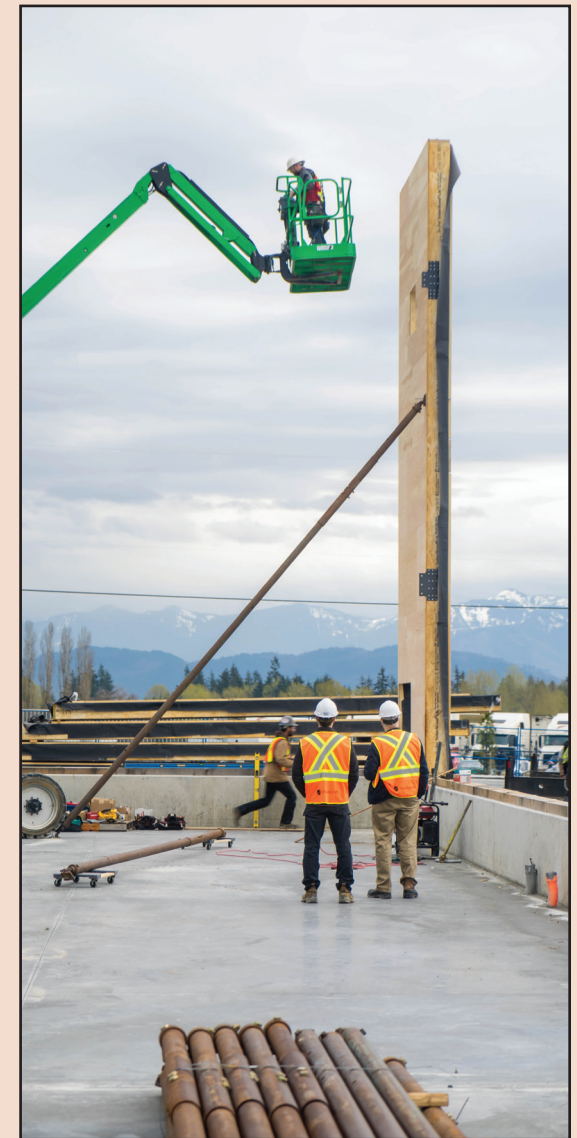
Fig. 4.6: Full-height wall panels
