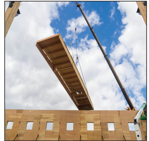
Fig. 4.4: Roof panel being lifted into place
