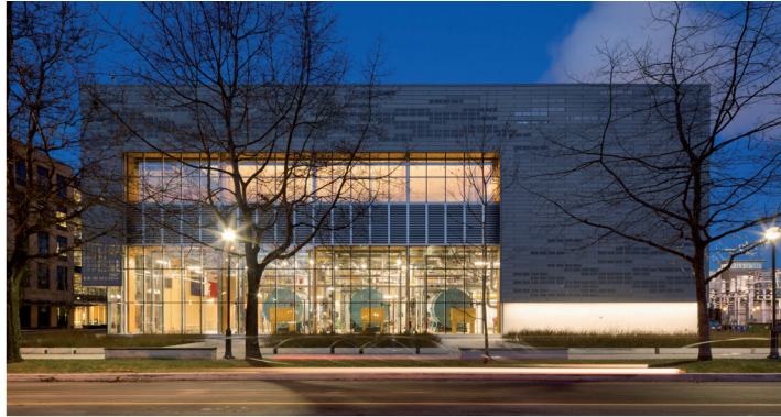
UBC Campus Energy Centre Vancouver, BC
