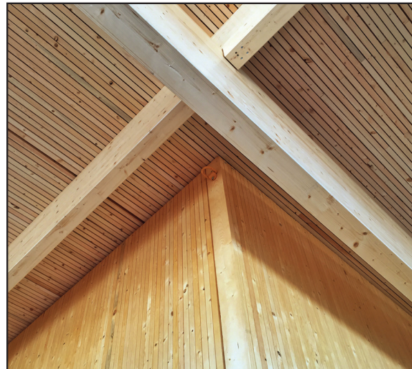
Fig. 4.14: DLT panels in the office area
