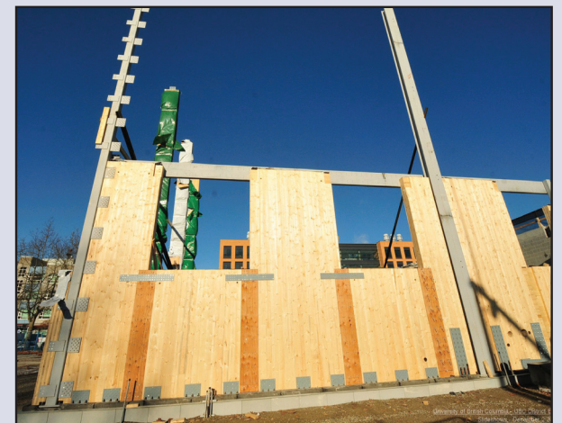
Fig. 3.9: CLT wall panels are stacked vertically and secured to the glulam frame
