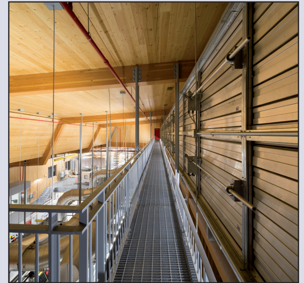
Fig. 3.8: The sloping roof also features structural CLT panels
