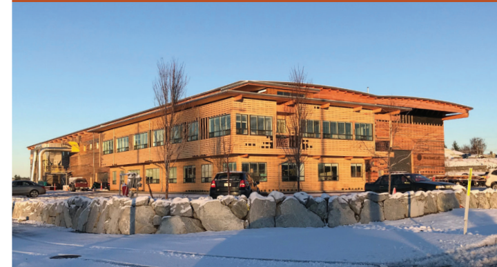
Fig. 4.1: Although they appear to be a single building, the office and factory areas are structurally distinct
