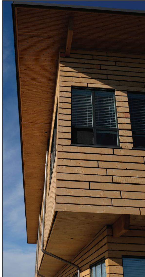
Fig. 4.16: The building is clad in a rainscreen system of unfinished Alaskan yellow cedar boards
