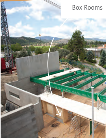
Roof Level: CTL Transfer Beam
