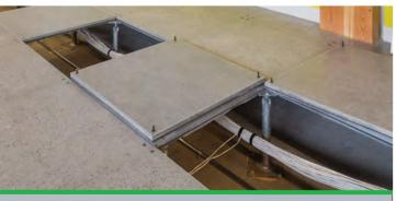
Access flooring. For a building of this size and type, the concealed space must be non-combustible. *Photo: KK Law, Courtesy: naturally:wood*
