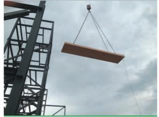
Floor panels were lifted into place by crane Courtesy: Proscenium Architecture
