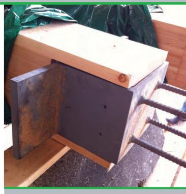
The columns have end-to-end bearing to minimize shrinkage over the height of the structure. Rebar rods on the saddle connector fit into holes drilled in the base of the column above. *Courtesy: Fast + Epp*
