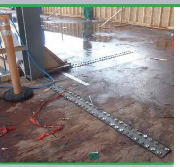
Steel strap tying wood floor to steel frame for lateral bracing Courtesy: Fast + Epp
