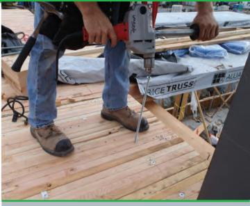
Once in place, the floor panels were lag screwed into the glulam beams Courtesy: Proscenium Architecture
