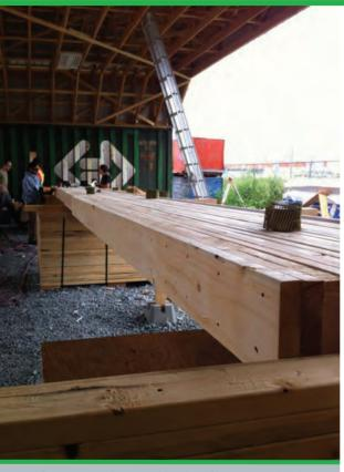
The floor construction resembles that of late 19th and early 20th century commercial buildings across Canada. This technique is being revived and updated to reduce the environmental impact of new buildings. *Courtesy: Fast + Epp*
