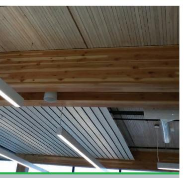
Small gaps were filled with mineral wool insulation and sealed with fire-rated caulking to meet fire separation requirements. Oversize gaps also had wood filler strips nailed in place from below. *Courtesy: Ventana Construction*
