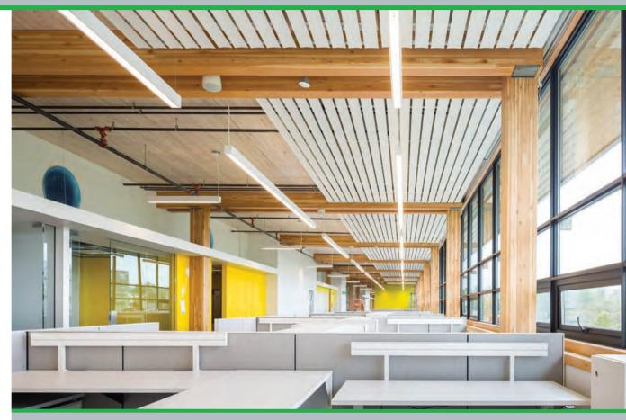
Radiant ceiling panels are positioned alongside the windows to provide additional heating or cooling as required *Ed White Photographics*
