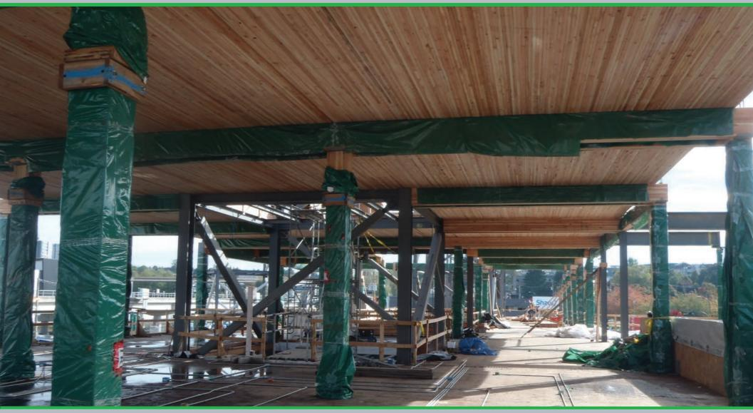
The nail-laminated floors are tied into braced steel frames that provide lateral resistance to the structure Courtesy: Fast + Epp
