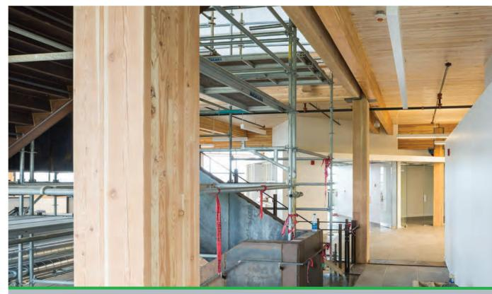
The dropped beams around the perimeter of the atrium are designed to contain smoke in the case of a fire *Photo: KK Law, Courtesy: naturally:wood*
