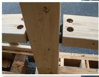
The structure is designed with simple connections to be completely demountable, enabling the material to be recovered for future use with no loss of structural value.
