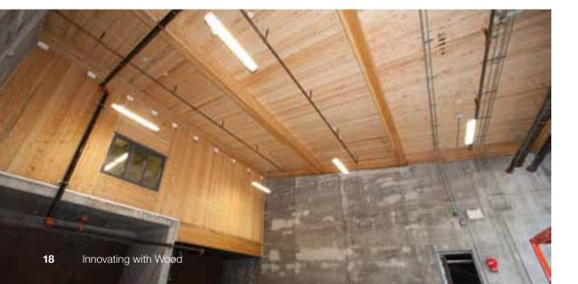
The introduction of CLT panels to North America provides architects and engineers with more design options and a more sustainable building system for heavy structures; one that displaced applications normally relegated to concrete or masonry. This highly promising wood system has been identified by the forest products industry, as well as the research and design communities, as a new and innovative opportunity for advancing wood in non-traditional applications.
