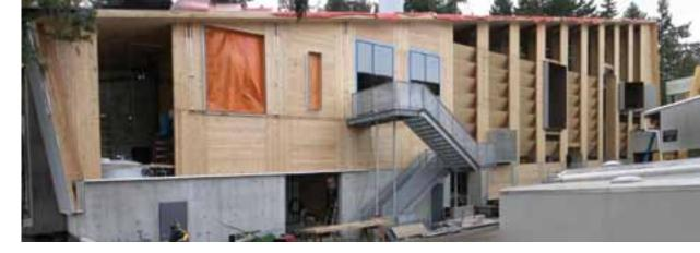
design, and showed air intake on the low windward side, and air exhaust on the high leeward side. As well, horizontal, outwardly angled CLT panels helped direct heat upwards and away from the power plant towards the glazed areas where heat could be conducted to the exterior. These panels also encouraged a convective flow to mitigate the formation of condensation on the glazing.
