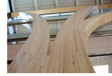
A third party consulting company with expertise in building code and fire protection was hired to develop a proposal for an alternative solution to demonstrate, through the use of empirical data, that heavy timber (glulam) could be used throughout the atrium. In the end the atrium consisted of heavy timber and acted as a separation between the existing building and the new development at the third-storey. The glulam was supplied by Western Arch Rib (Manitoba).
