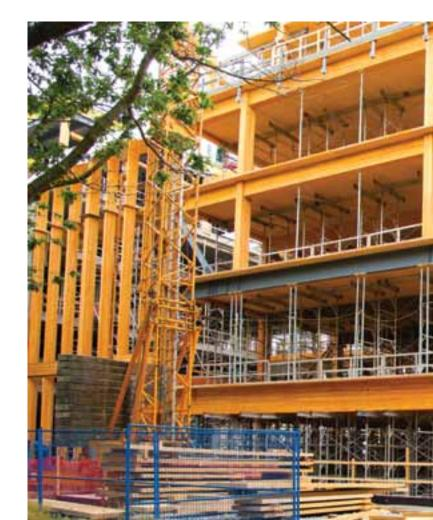
The combination of solid, cross-laminated wood and woodconcrete composite panels make the academic wing of the UBC ESB an innovative project in Canada – raising the bar for the use of wood in large scale, high performance projects. Glulam, LSL, CLT components and connectors were supplied through Structurlam Ltd, of Penticton, BC. Weyerhaeuser produced all of the LSL panels for the project.
