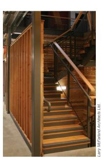
was placed on the selection of indigenous species for finishes and for structural applications, including western red cedar, which has a strong historic and cultural importance in coastal British Columbia. Cedar slat walls, comprised of 1 x 4 boards, were used to define the enclosure around the central stair, and to add emphasis to walls in other rooms.
